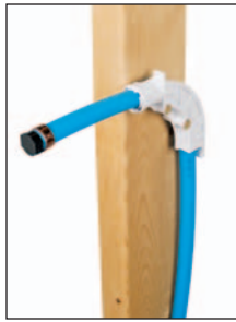
One 525-P2 nailed directly to the stud.
